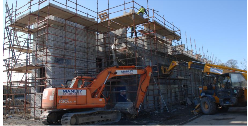
Mid-Way through deep retrofit
