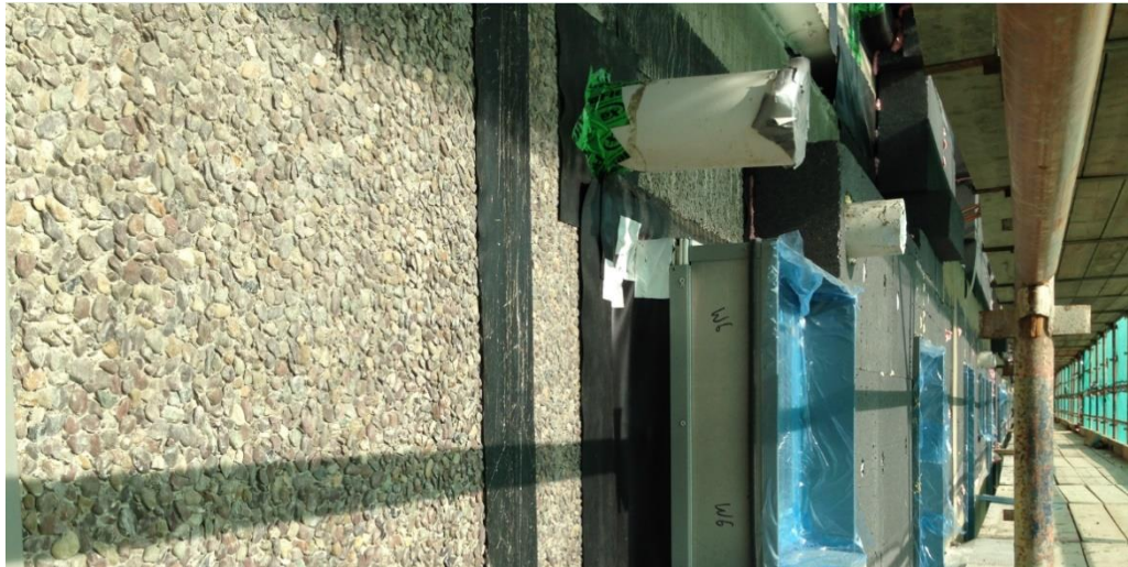
External wall detail with ventilation duct
