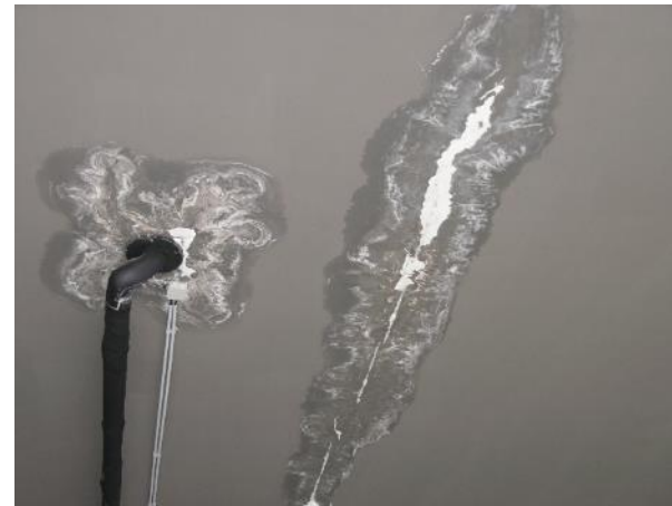
Insufficient roof slope for adequate water drainage
