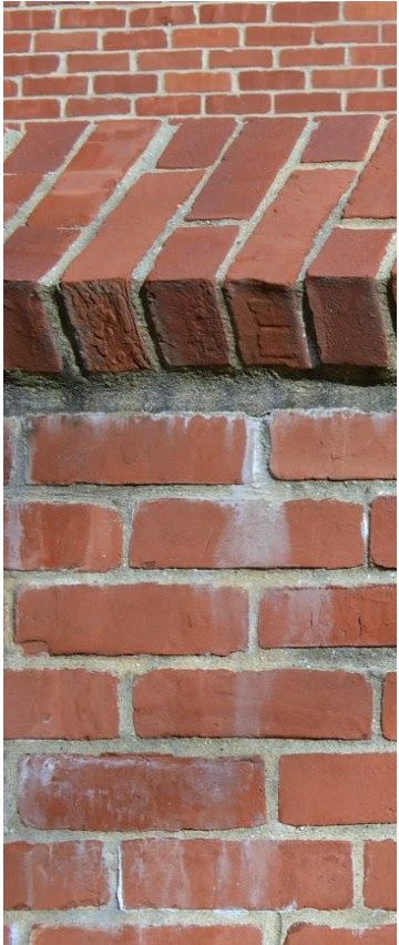
Unplastered brick or block
