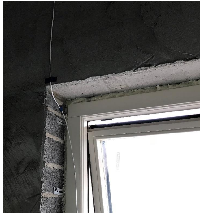
Window to wall connections
