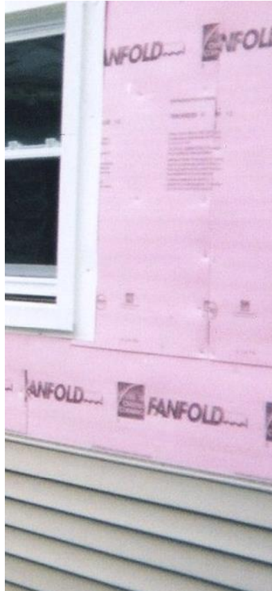
Insulation boards & tongue & groove cladding
